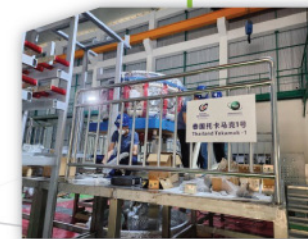
TT-1 Installation @ TINT Ongkharak
